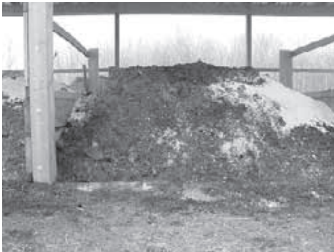
Figure 8: This bin has a concrete base with a 4 in. curb. Courtesy: Birch Bay Pork .
